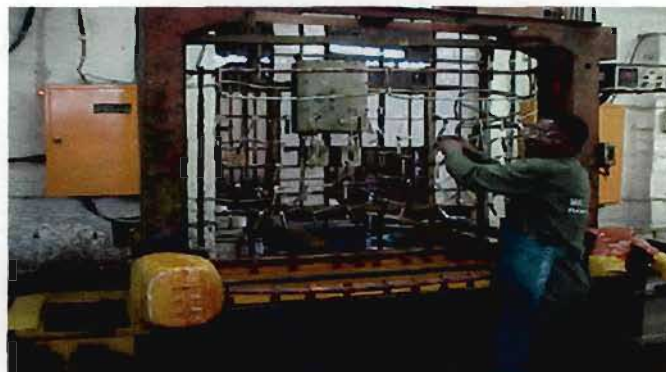
Figure 3.4 Gantry used in lifting jigs in and out from chromium plating bath
