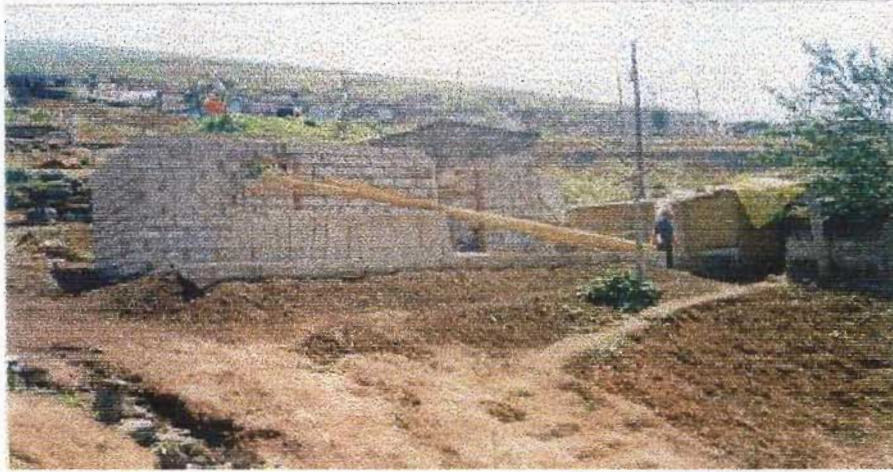
Figure 4.11 A house under construction
