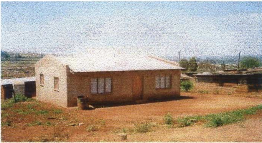
Figure 4.12 and 4. 13 Four-roomed housed in Thembalihle built with help from Agishana
