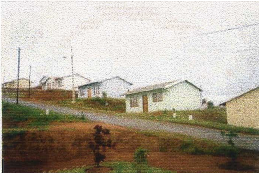
Figure 4.7 Houses at Pioneer Park also showing the slope
