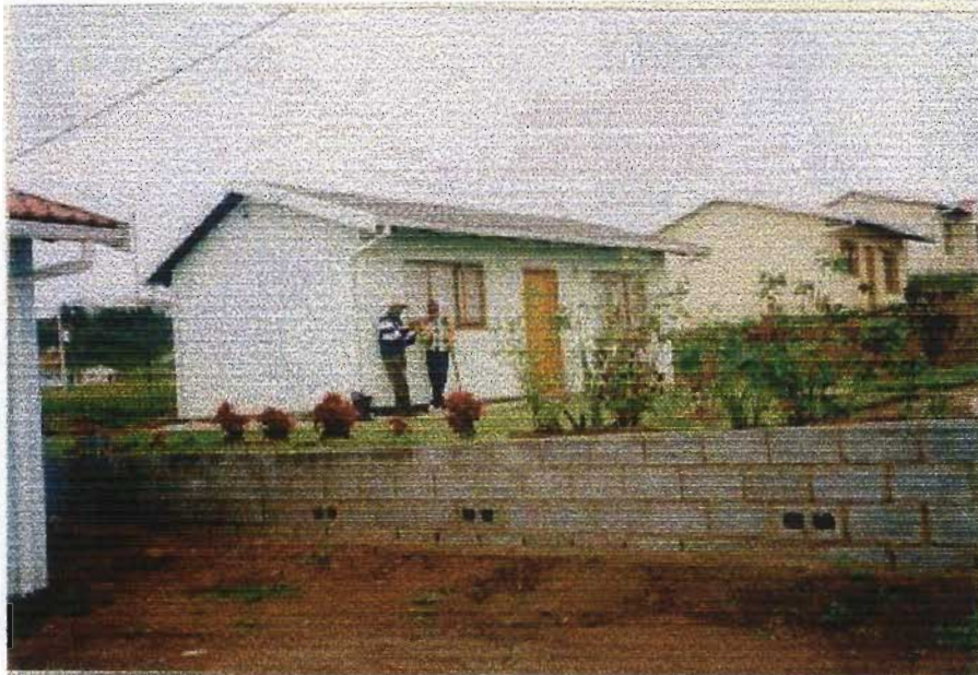
Figure 4.6 A House at Pioneer Park with Retaining Walls
