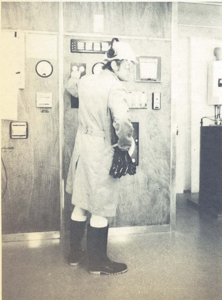
View of the control panel.
