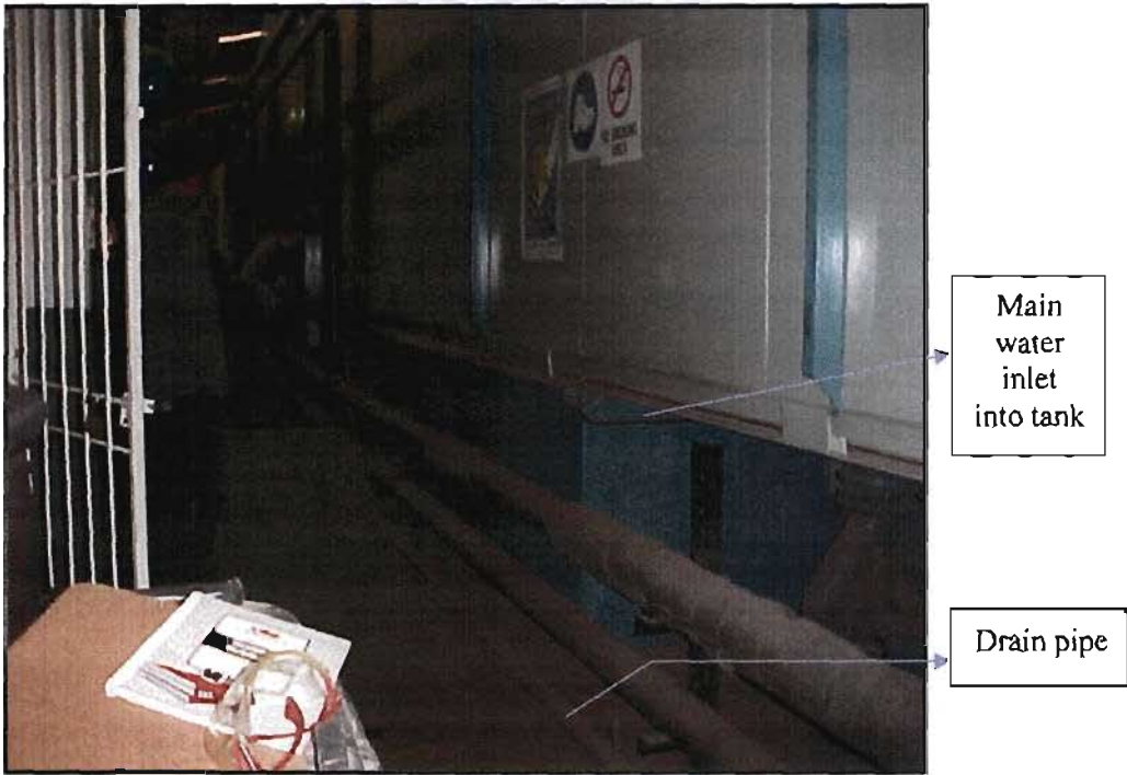
Figure 4.14 Main pipe inlet into Tank 2
