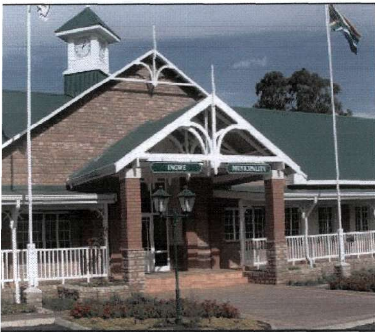
Plate 5.2 : New Ingwe Municipality offices and station
