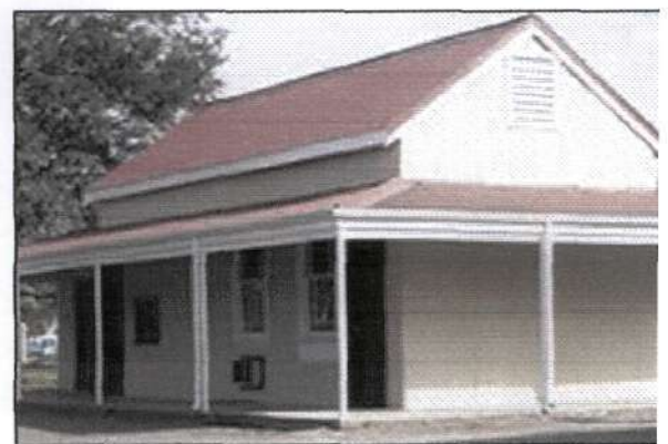
Plate 5.3: Coffee station – restored old station
