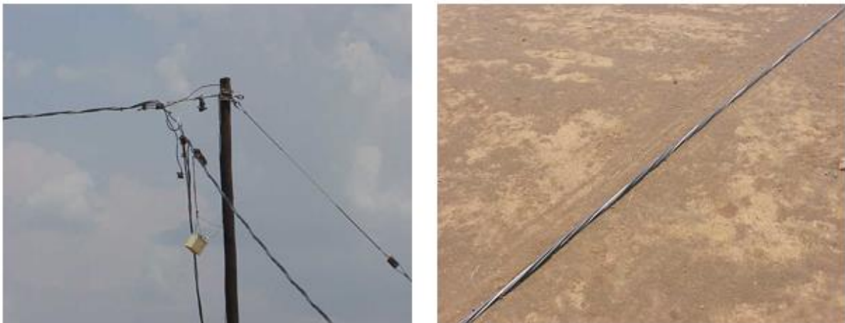
Figure 2.8 Broken conductor after being hooked by a truck at Skhunyani village
