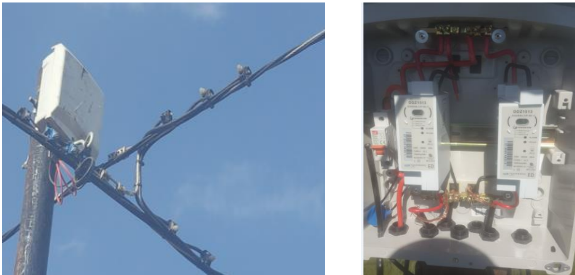
Figure 3.3 and 3.4 Service Pole Top Box
