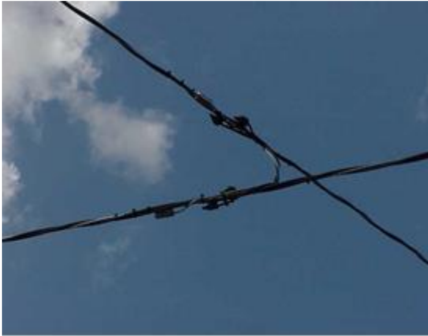
Figure 2.6 Flying jumpers connection on aerial bundled conductors
