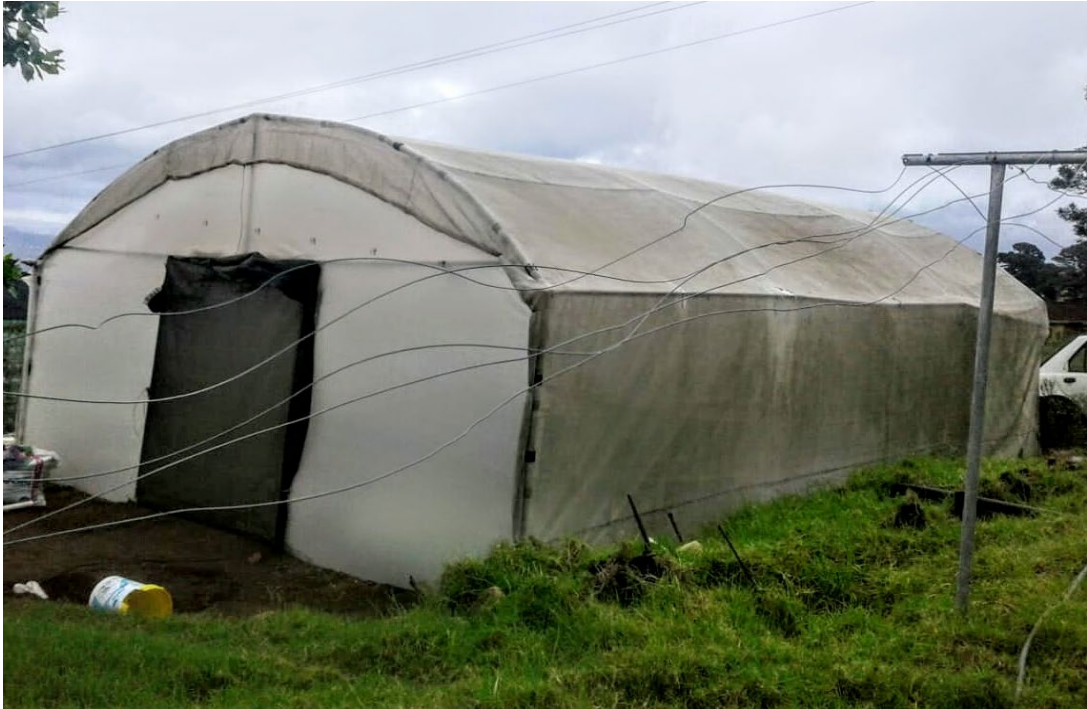
Figure 4.3 Ndwedwe aquaponics tunnel infrastructure
