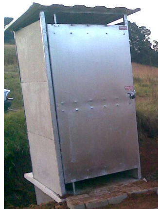
Figure 4-29: Prefabricated toilet structure
