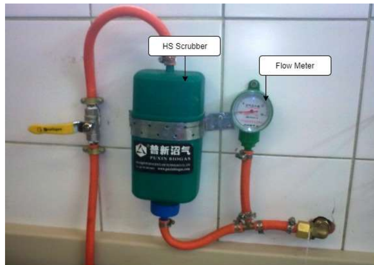
Figure 4-24: Example setup of H 2 S scrubber and flow meter
