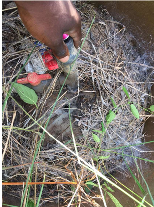
Figure 4-3: Damage to dome gas outlet valve fitting
