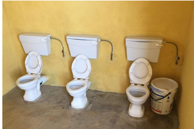
Figure 4-27: Water closet toilet systems at Vukuzenzele ECDC
