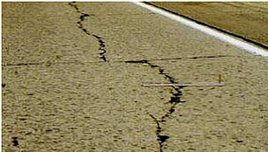
Plate 2- 2: Corner fissures in concrete pavements (after Pacheco-Torres et al., 2018).
