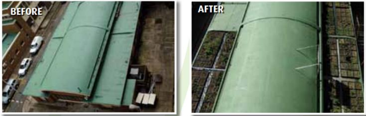
Figure 2-11: eThekweni pilot green project before and after construction.
