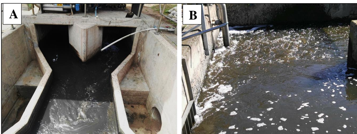
Plate 4. 7 Durban wastewater treatment plant, A): - Influent, B): - Effluent. Coordinates: - Umhlathuzana S 29°52'32,5 E 29°52'32,5".
