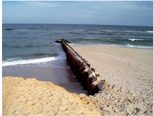
Figure 2.16: Temporary timber groyne illustrating transport direction from right to left of image
