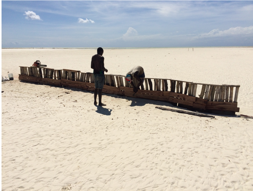
Figure 4.10: The voids of Groyne 1 created from the skewness of the vertical supports. Source: Author
