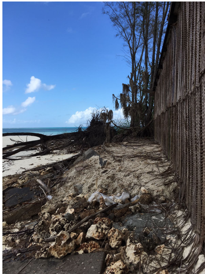
Figure A.2: May 2017 South Eastern corner of Mnemba Island. Complete loss of concrete floor slab
