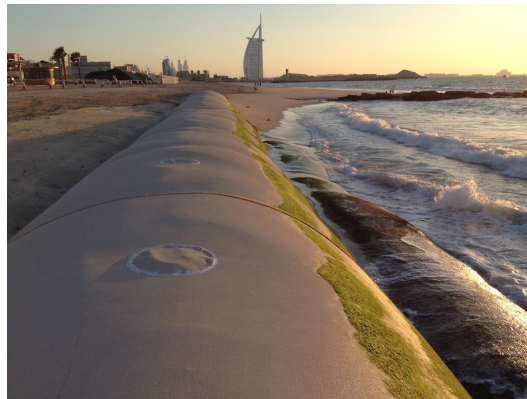
Figure 2.24: Geotube beach protection in DUBAI. Source: (PTSA, 2016)
