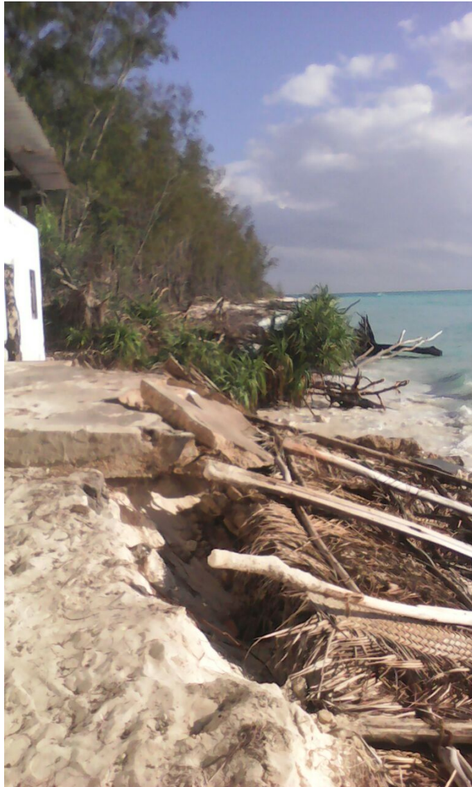
Figure A.1: 20 October 2016 South Eastern corner of Mnemba Island. Further collapse of concrete floor slab
