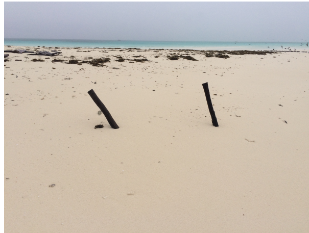
Figure 4.15: Groyne 2 status one day after construction.
