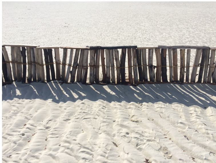
Figure 4.9: The voids of Groyne 1 created from the skewness of the vertical supports. Source: Author
