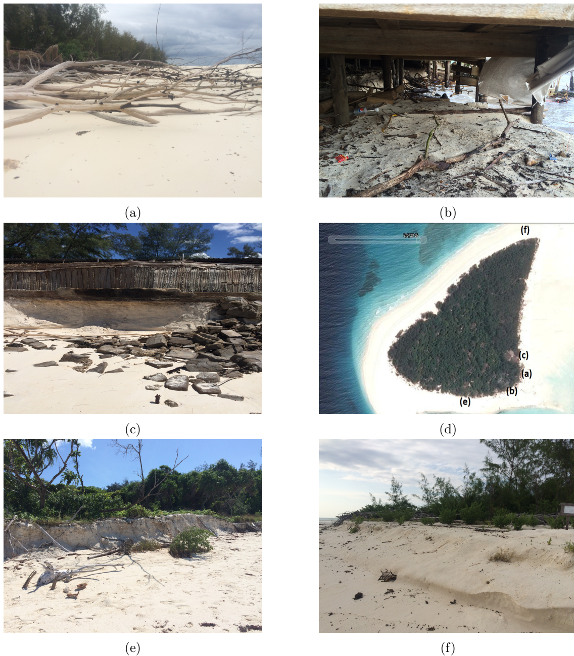
Figure 3.3: Erosion state as of 20 May 2016.(a) Fallen Casuarina trees. (b) Erosion undermining structures.(c) Collapsed floor slabs.(d) Image locations (Not to scale).(e) Beach scarp southern Bank.(f) Beach scarp northern Bank.
