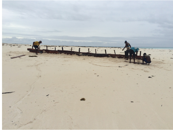
Figure 4.13: Groyne 2 at north-east corner
