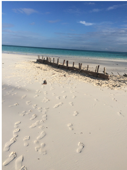
Figure 4.14: Groyne 3 at south-east corner.
