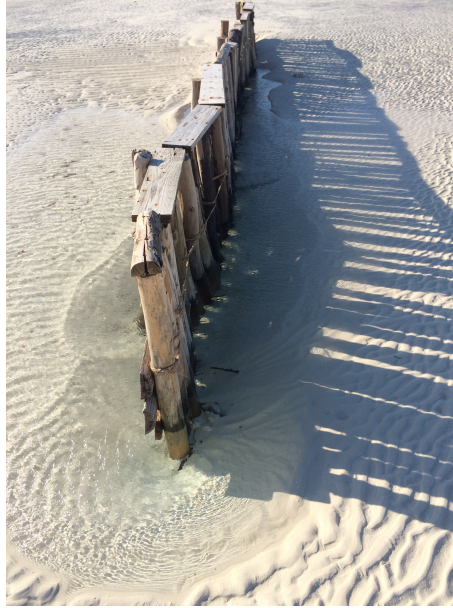
Figure 4.11: 30 May 2016, similar erosion pits on both landward(left) and seaward side of structure expected from periodic flooding and drying by tides. Source: Author
