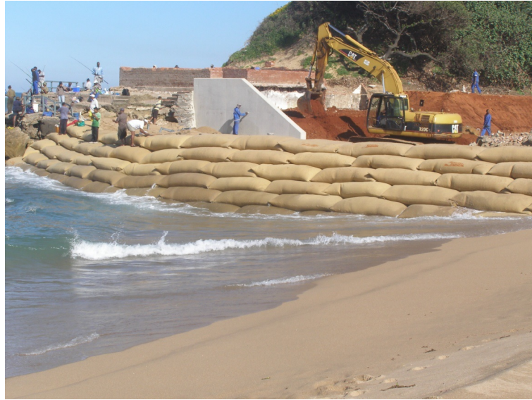
Figure 2.26: Geocontainers used for protection against wave action and erosion on Isipingo Beach, KwaZulu-Natal. Source: (Kaytech, 2016)
