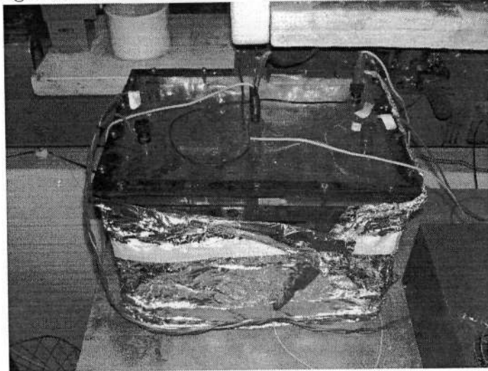
Figure 5.16: Photo of the high-voltage transformer
