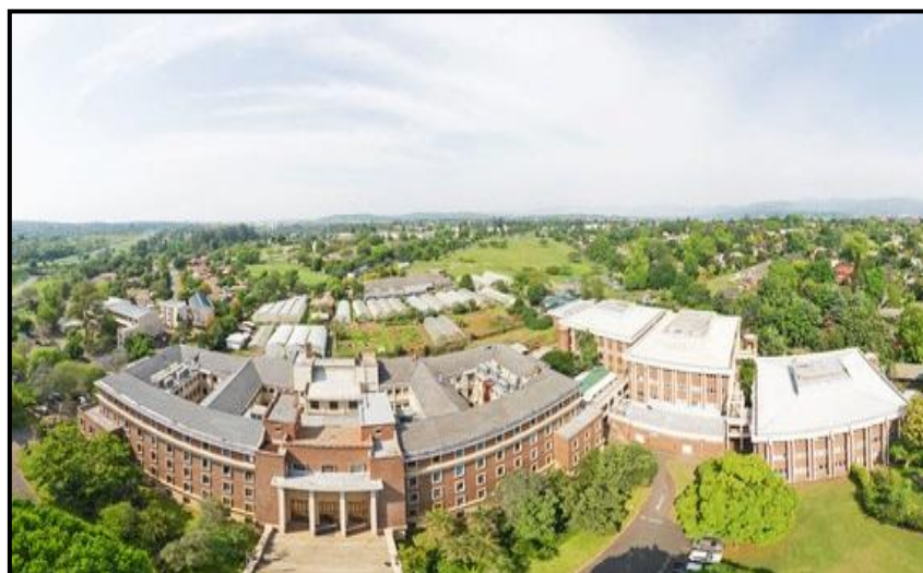
Figure 3.2 Ariel view of the Rabie Saunders Building on the Life Sciences campus, Pietermaritzburg
