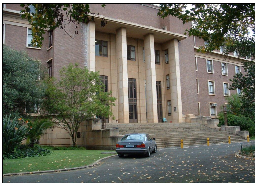
Figure 3.3 Entrance to the Rabie Saunders Building
