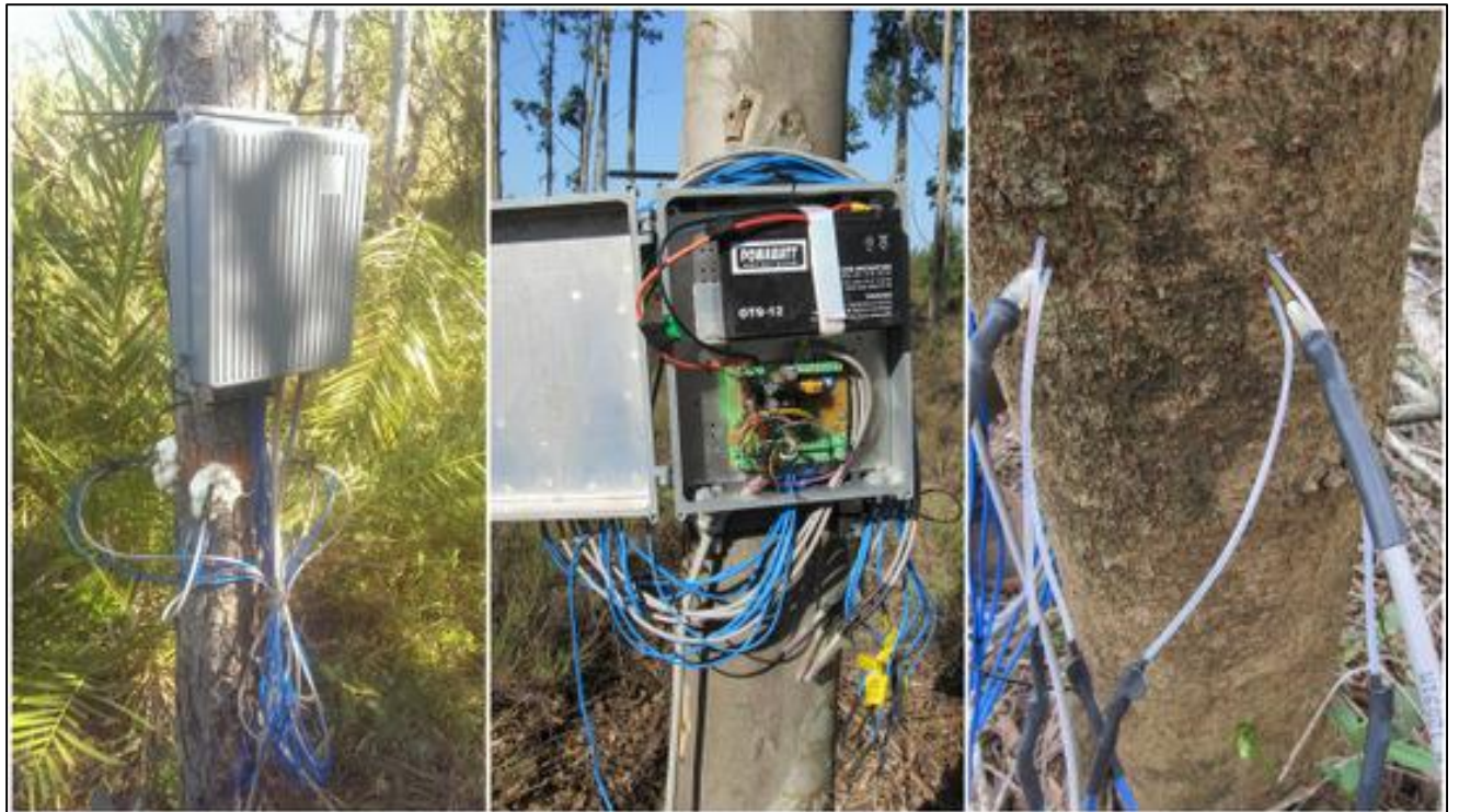
Figure 3.8 The new heater box enclosure and probes
