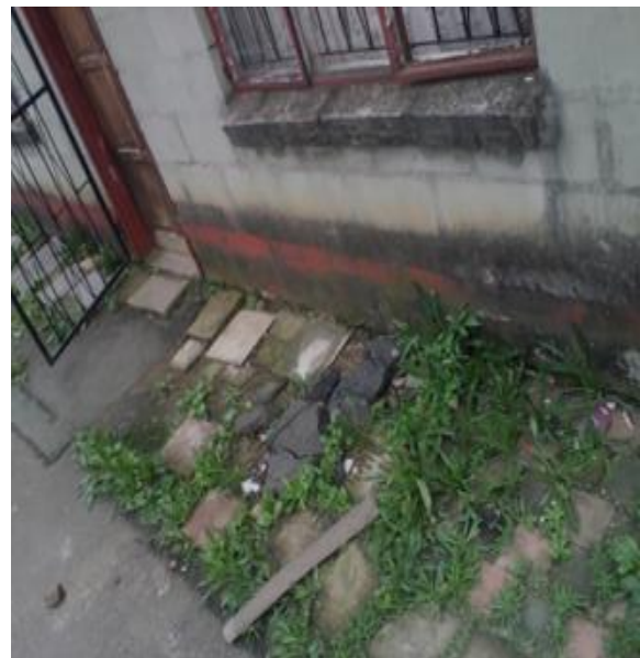
Figure 5.5: Damp on Walls
