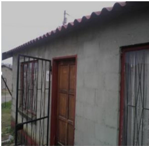
Figure 5.4: House Showing Unavailability of Gutter
