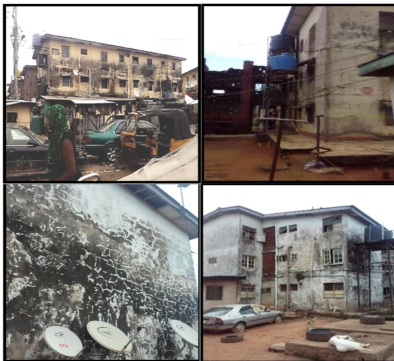
Plate 7.3 Poor House Painting Condition in Public Low Income Housing Estate
