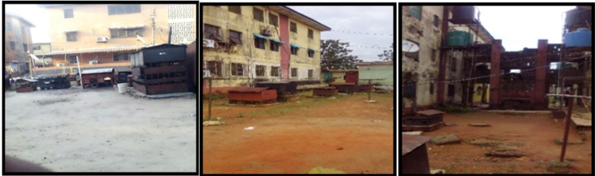
Plate 7.5 Generator as Alternative Source of Power Supply in Housing Estate
