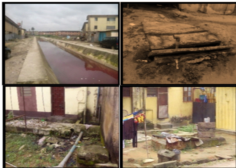
Plate 7.12 Different Sewage Conditions across the Housing Estate
