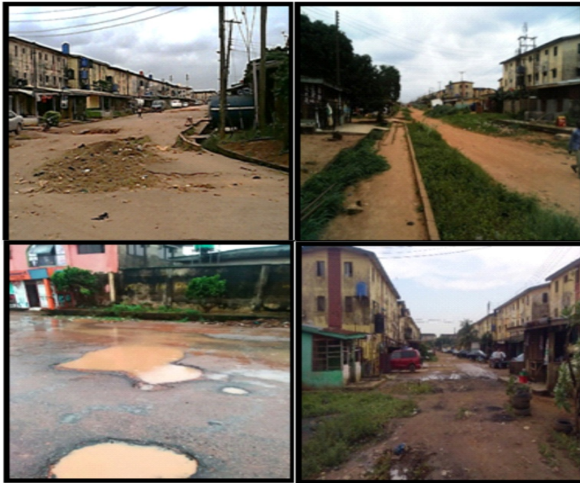
Plate 7.7 Deplorable Road Surface Condition across the Estates
