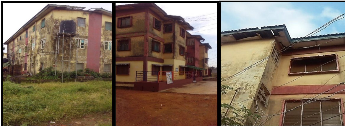
Plate 7.2 Poor Roofing and Ceiling Conditions in the Estate.
