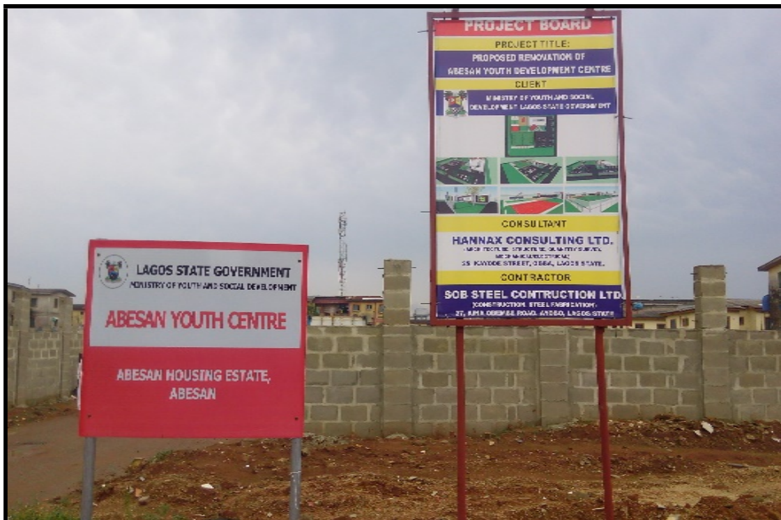
Plate 8.1 Site of Skill's Acquisition Centre in Abesan Public Low Income Housing Estate
