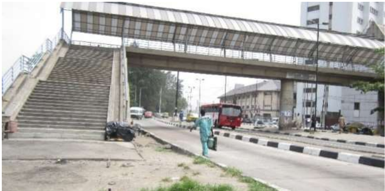
Plate 25: Pedestrian bridge located at CMS and pedestrians seen not using the pedestrian footbridge at Apongbon
