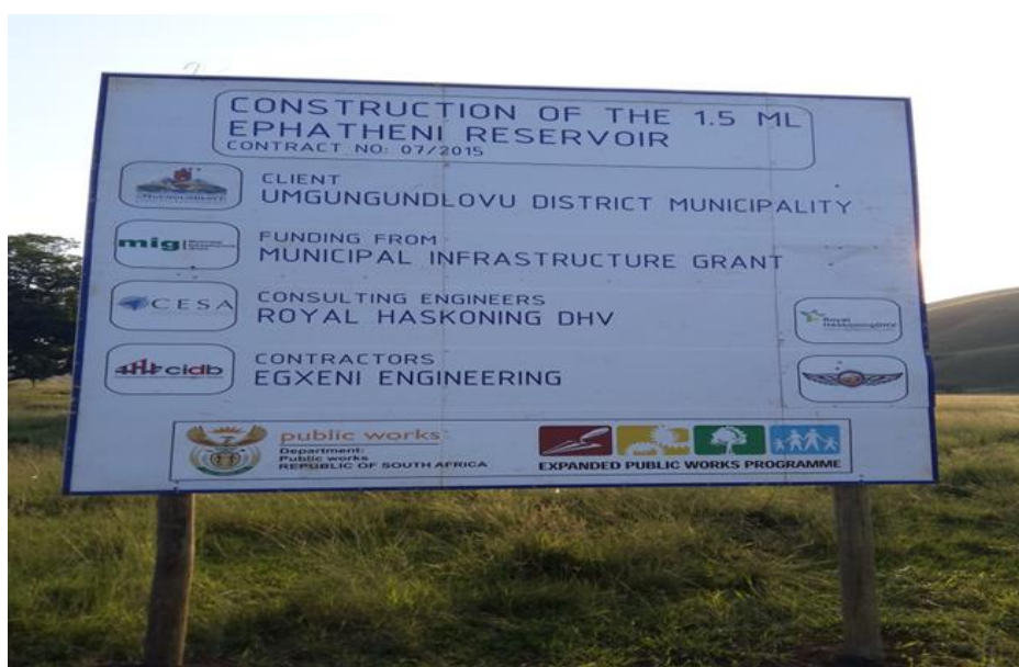
Figure 11: Construction of the Phatheni reservoir
