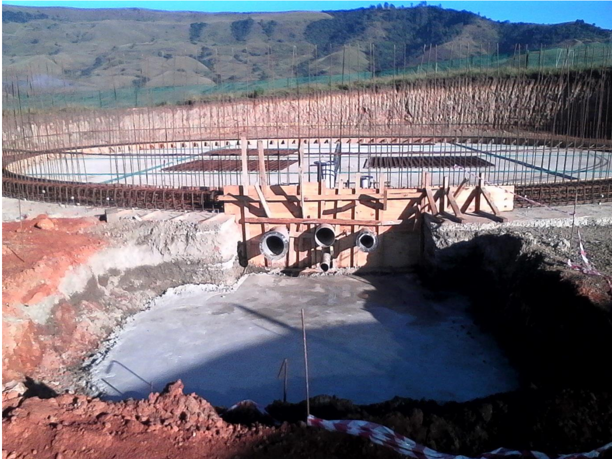
Figure 14: Picture depicting unfinished construction of the reservoir
