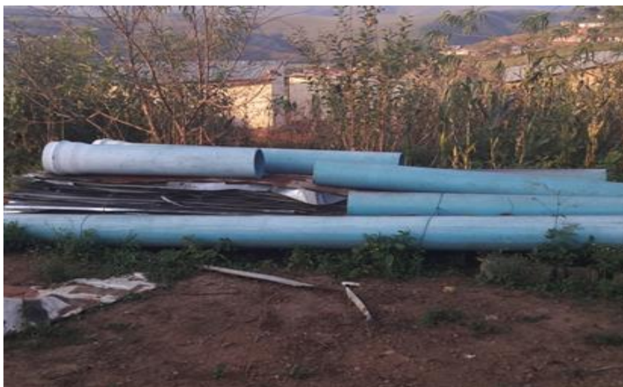
Figure 10: Underutilised water pipes from the unfinished water project undertaken in Phatheni
