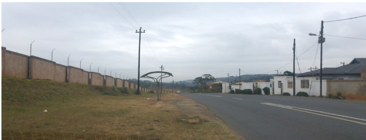
Plate 4.15: Rural-Urban Divide (Cotswold Downs perimeter wall on the left, Embo on the right)
