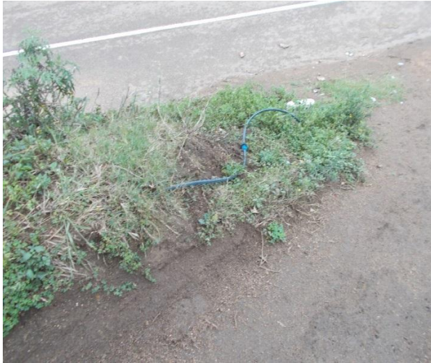
Figure 8: Exposed Water Pipe
