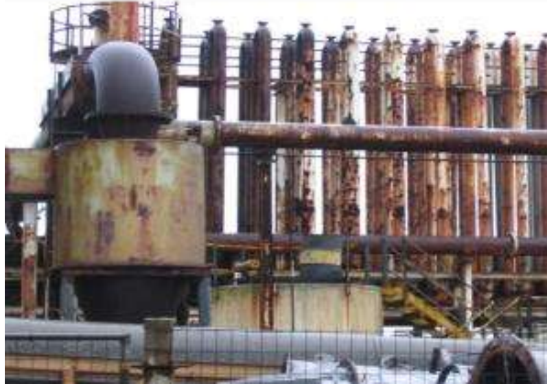
Figure 5.2.3: The abandoned remains of the Thor Chemicals Factory. Source: The Mercury, 2012
