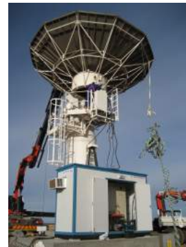
(c) Mounting the assembled primary reflector onto the base.
