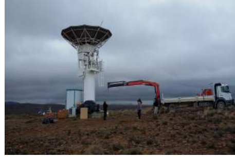
(b) The operational southern system at the MeerKAT support base, Klerenfontein, South Africa.
