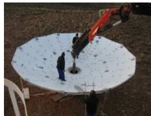
(b) Lifting the assembled primary reflector with a crane.
