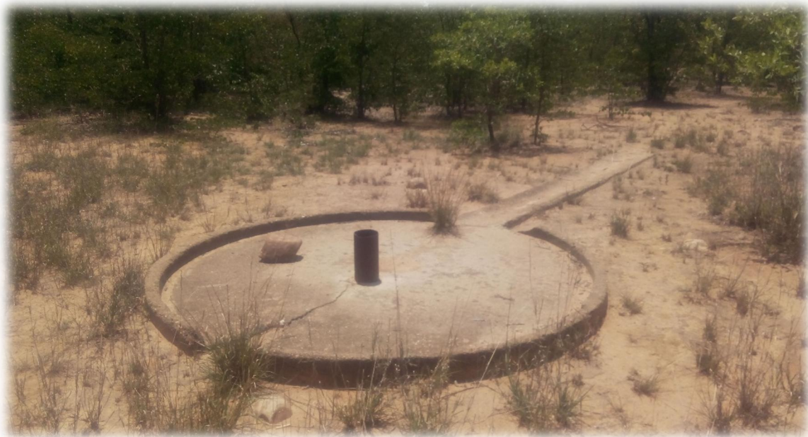
Figure 4.1: A dilapidated borehole in Village one, Ward 11 of Mhondoro-Ngezi District (Photo by author)
