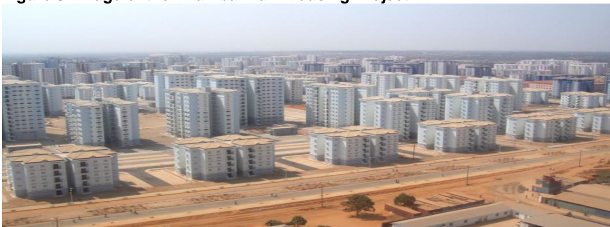
Figure 3: Image of the Kilamba Kiaxi Housing Project
