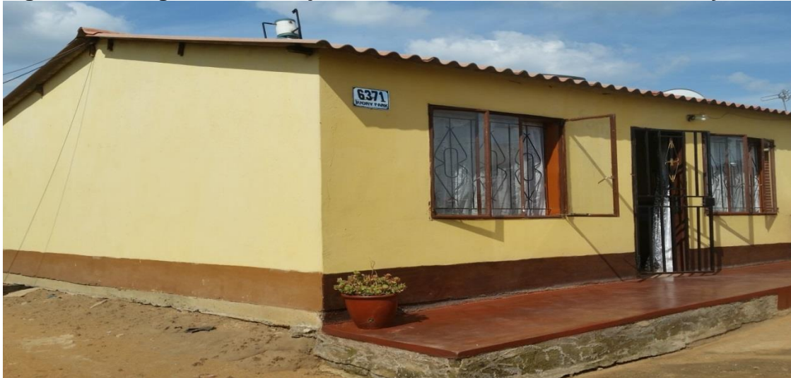
Figure 14: Image of NYB Project house installed with extra security features
