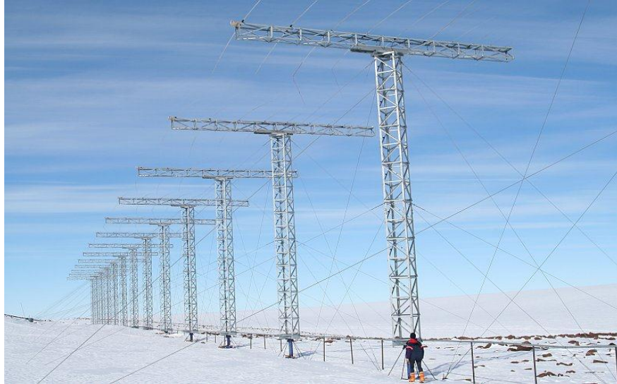
Figure 3.4: The SANA E 16 antenna array.
