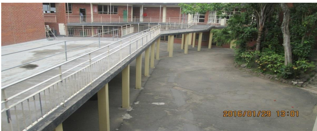
Figure 5.12 View of the quad and how classrooms open up to it
