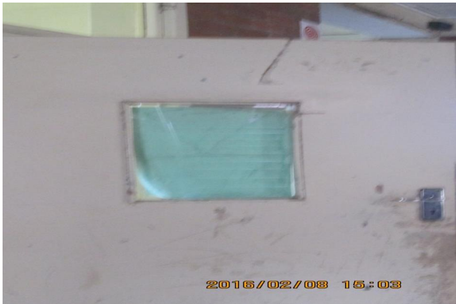
Figure 5.14 Door with a sealed glass panel at NHS
