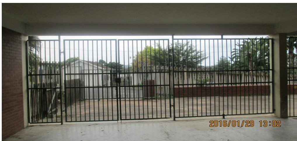
Figure 5.13 Gate locked during class time at NHS
