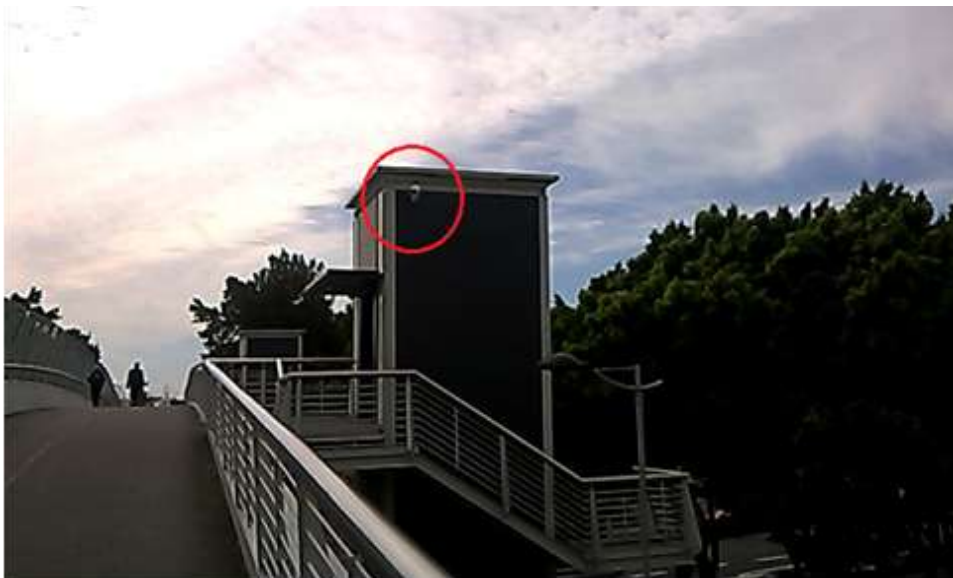
Plate 29: Overt use of CCTV (in red circle) on Canal Walk at North Wharf Square
