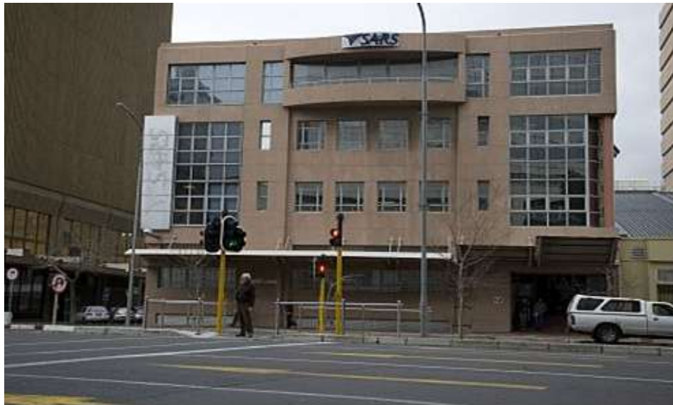
Plate 19: The South African Revenue Service (SARS) Building
