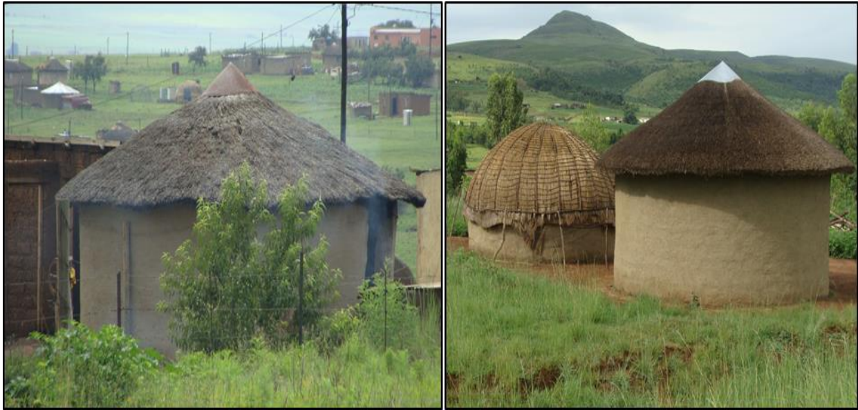
Figure 5.9: Rondavel structures used for cooking in Bergville (Author, 2016)
