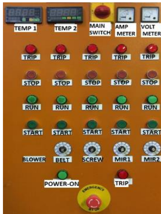
Figure 3-4: Control panel of the laboratory scale LaDePa
