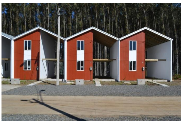
Figure 12: Villa Verde homes before user additions Image source: Cristian Martinez
