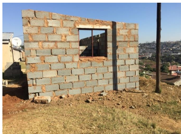
Figure 31: Poor quality block construction Image source: Author's own
