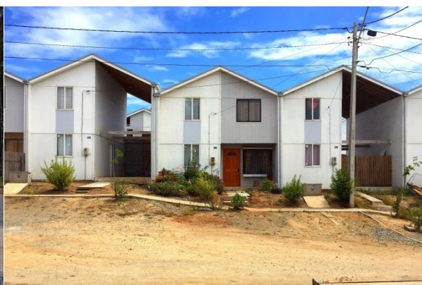
Figure 13: Villa Verde with user additions (center) Image source: Elemental
