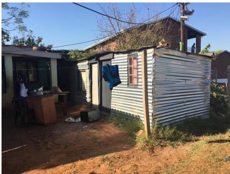
Figure 39: Informal additions to RDP house Image source: Author's own
