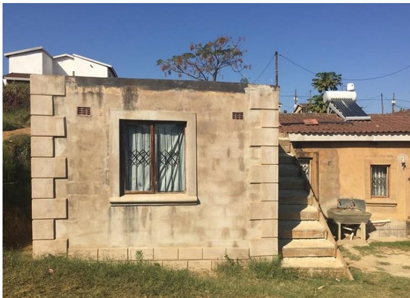
Figure 29: Self-erected stair to upper storey extension Image source: Author's own
