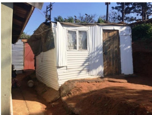
Figure 30: Unsafe metal sheeting construction Image source: Author's own
