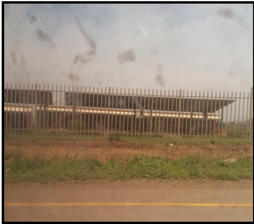
Figure 4.4 The almost complete taxi rank in Ntambanana Municipality
