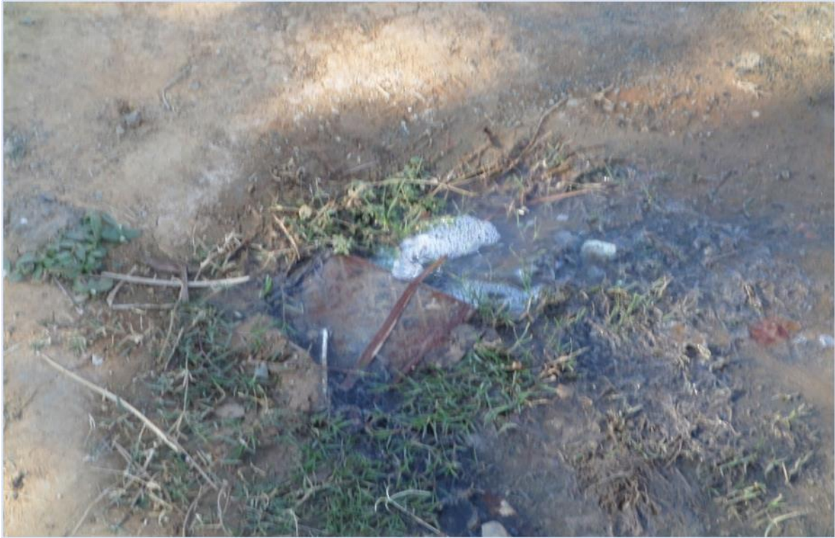
Plate 5.1: Leaking sewer pipe will cause health related flood risks ( Photograph by Njabulo Ngcobo, 2015 )
