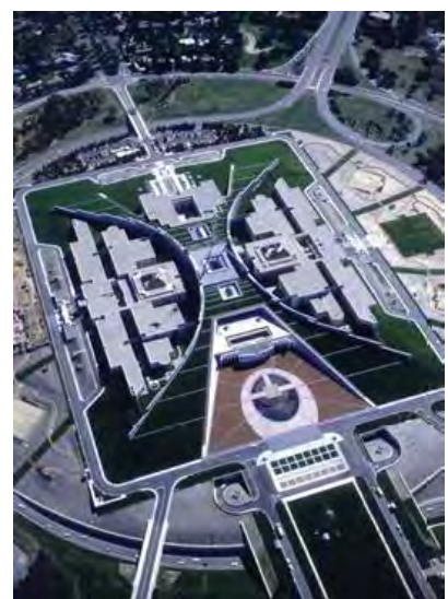
Plate 5-7 Aerial view of Parliament House before completion in 1988. Source: http://www.peo.gov.au/uploads/peo/docs/closer-look/CloserLook_Parliament-House.pdf
