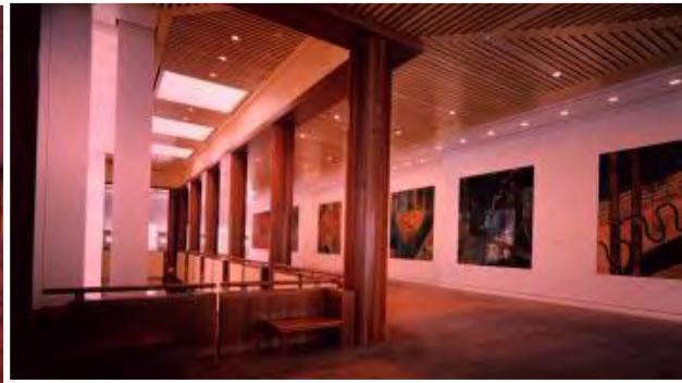
Plate 5-9 Top level showing the turpentine clad columns. Source: AR, volume 10, 1988: 57
