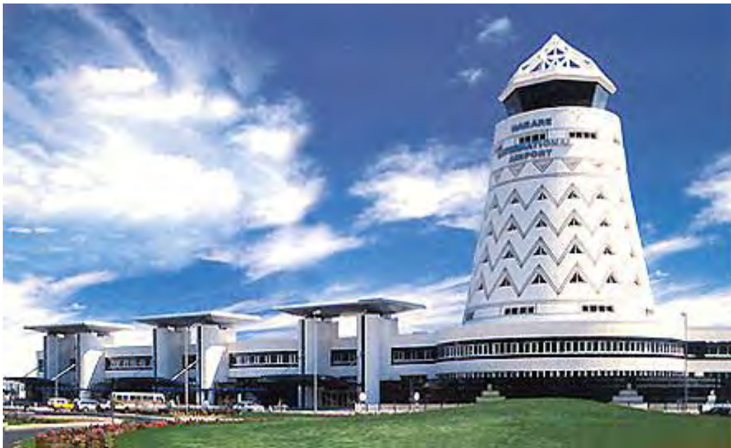
Plate 4-13 The new terminal at the Harare International Airport. Source: www.wikipedia.com
