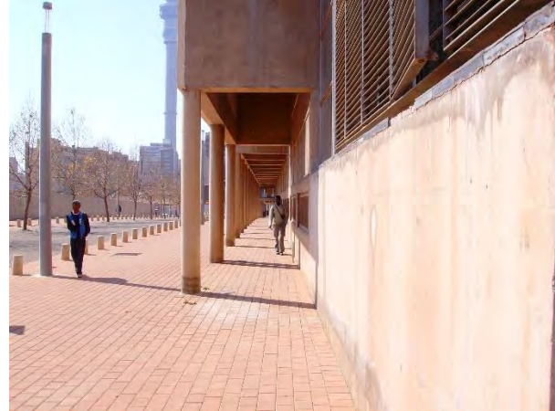
Plate 6-10 Image showing the typical materials used throughout the building. Source: Author
