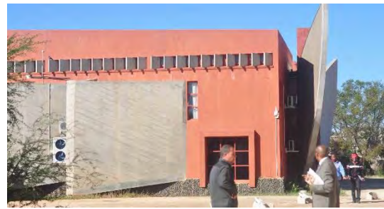
Plate 6-24 Partial south elevation of the Premier's Building. Source: Author
