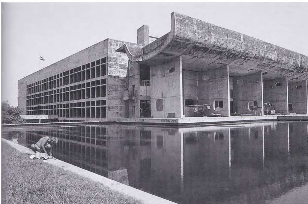
Plate 4-1 Chandigarh Legislative Assembly with bull horn shaped roof. (source: http://landlab.files.wordpress.com/2011/04/chandigarh-qt8.pdf )
