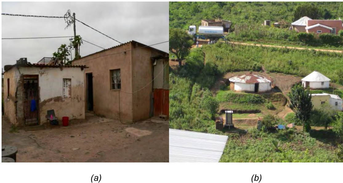
Figure 3-1 (a) A typical household with a VIP latrine in Besters, (b) A typical household with a UD toilet in uMzinyathi
