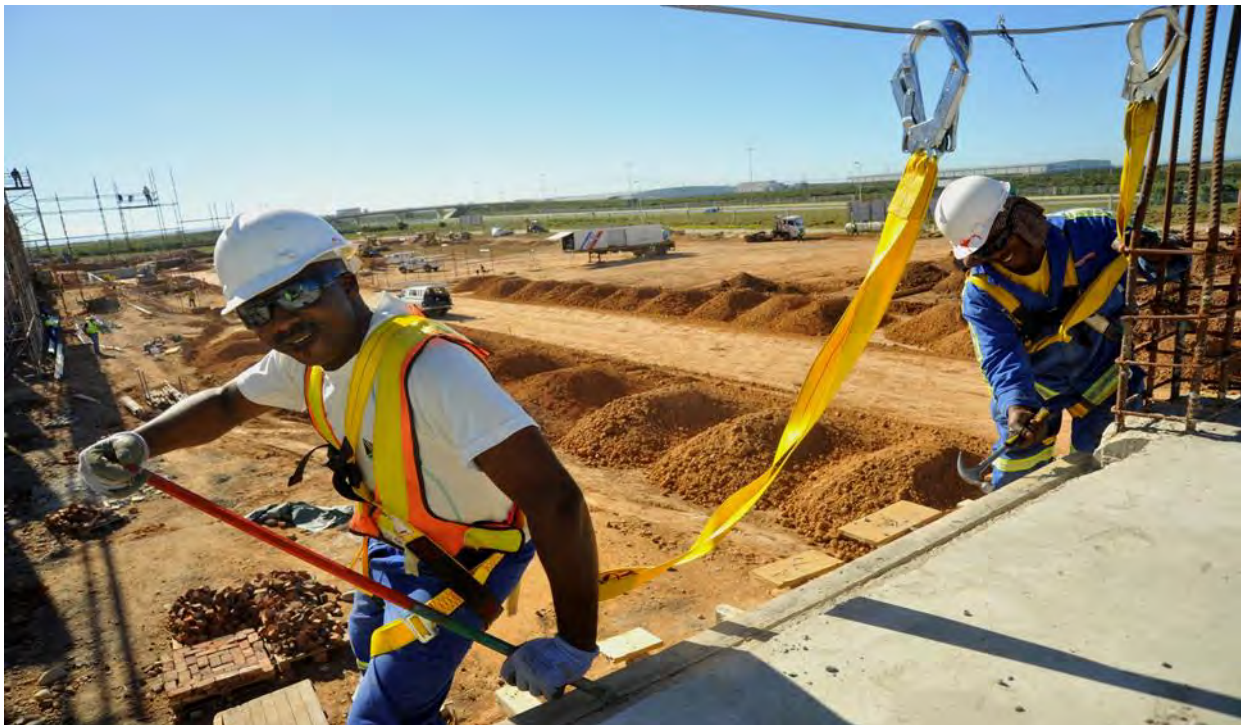
FIGURE 2-4 CONSTRUCTION SITE - COEGA
