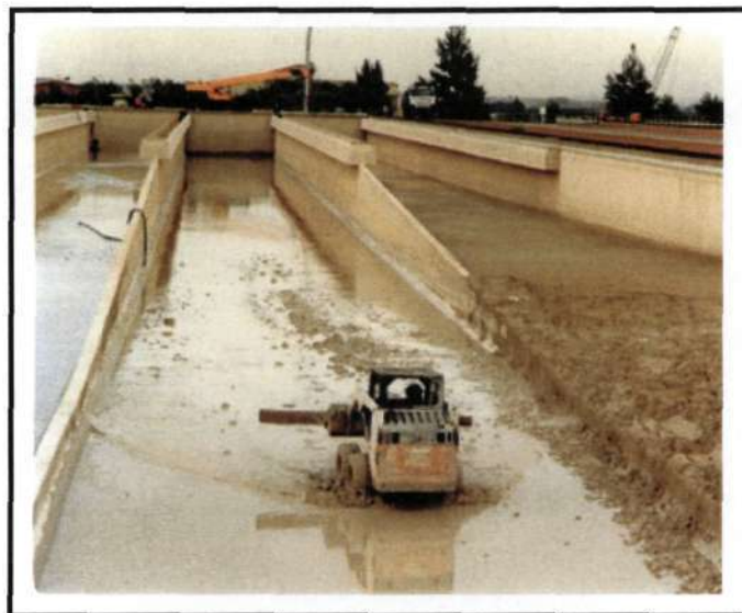
Figure 2.35: Removal of sludge from Rand Water's sedimentation tanks
