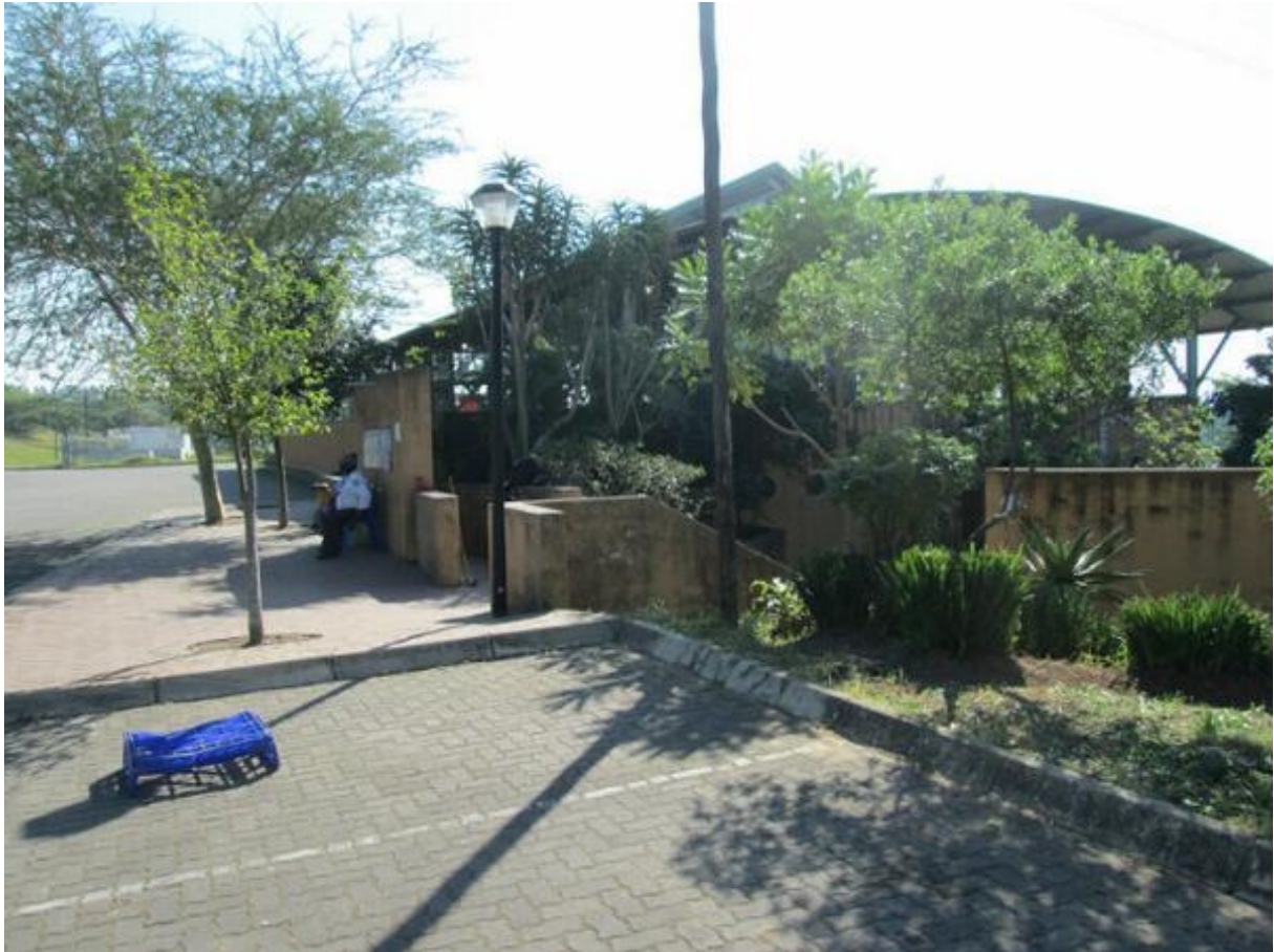
Figure 40: Image of the centre, currently, showing the need for building maintenance or lack thereof. (Photograph by author: 2015)
