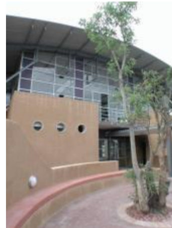
Figure 33: Image showing the central open plaza which links to various functions within the centre. (Source: http://www.equilibriumstudio.co.za/#!educationcommunity/c1se4 )
