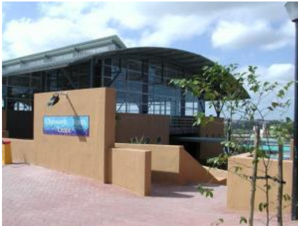
Figure 32: Image showing the main entrance off the top of the site located next to the main parking area. (Source: http://www.equilibriumstudio.co.za/#!educationcommunity/c1se4 )
