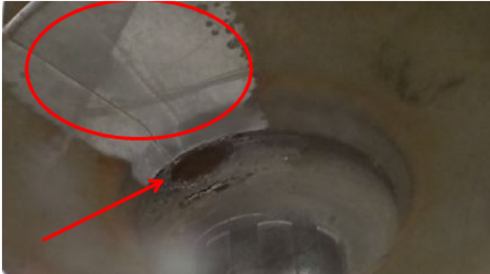
Figure 2.9: Burnt insulator fitting with sheath damage
