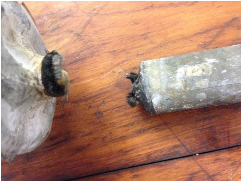
Figure 2.10: Severed end fitting as a result of arcing damage
