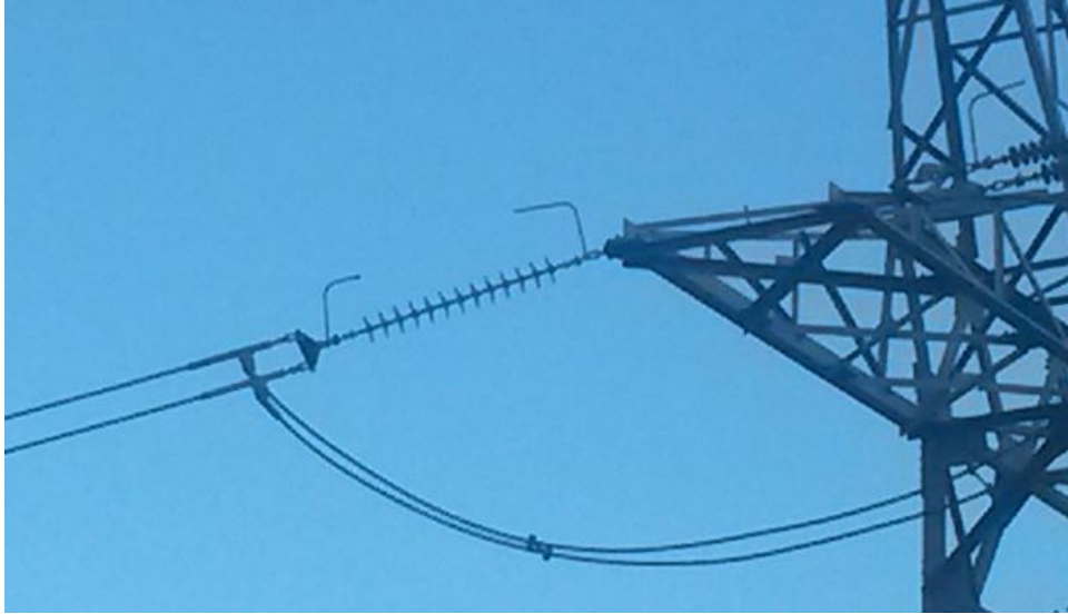
Figure 2.1: Arcing horn arrangement on a 132kV transmission line near substation
