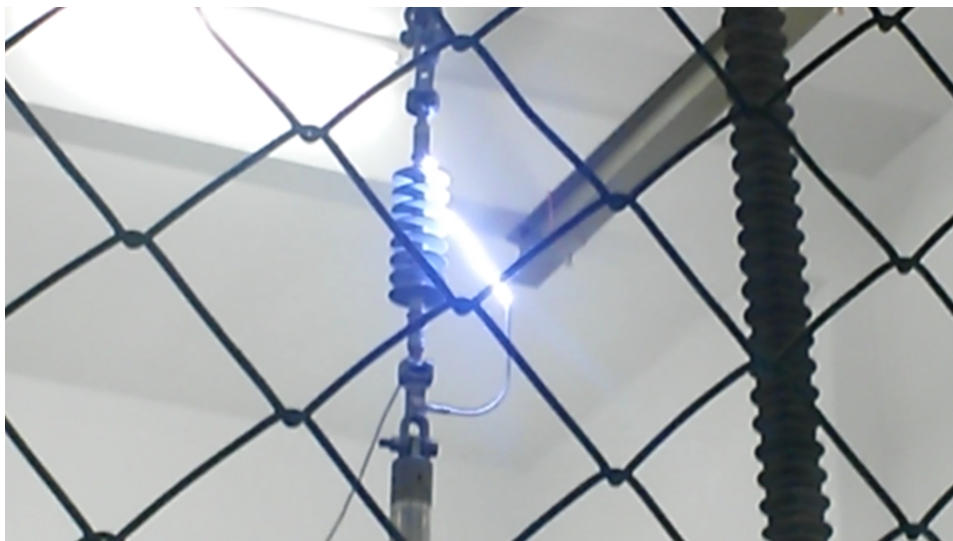
Figure 3.12: 22kV insulator flashover for one arcing horn to the fitting
