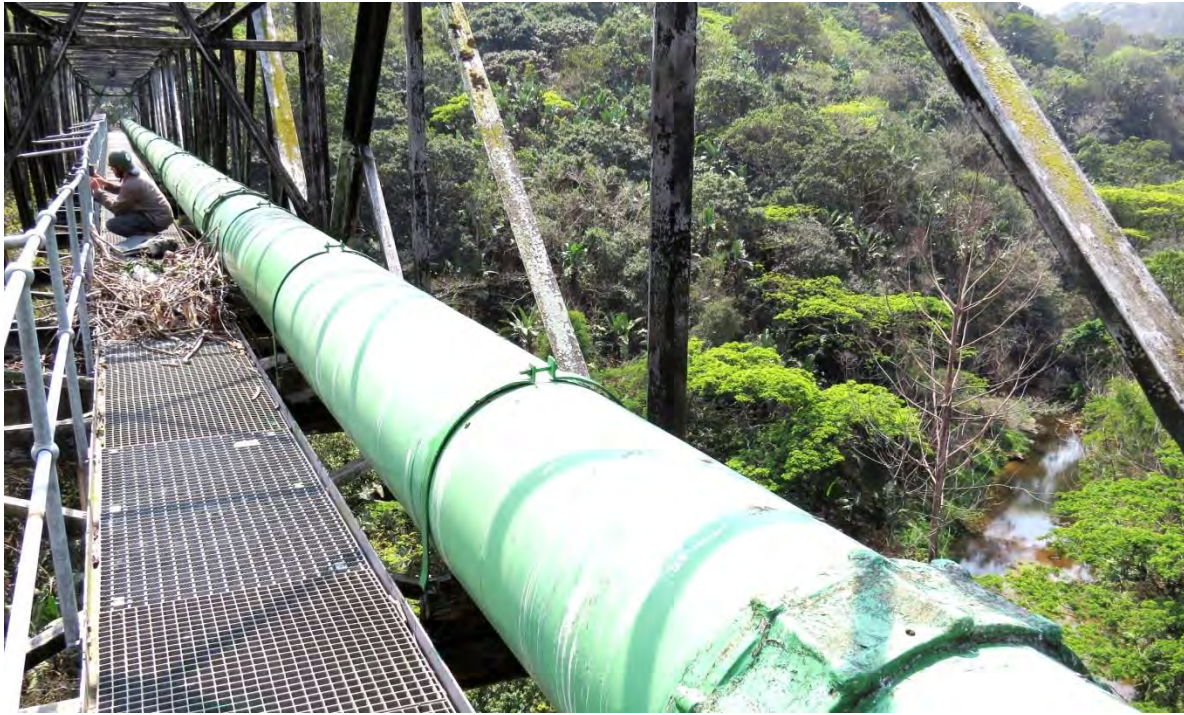
Figure 5.2 The first crowned eagle nest recorded on a human-made structure. SCM installs a monitoring camera, the eagle successfully fledged in Jan 2015. The nest is centred above the bridges' single support pylon, rising from the Umbilo rivers edge, Durban, South Africa. Photo credit Adam White, 2014.
