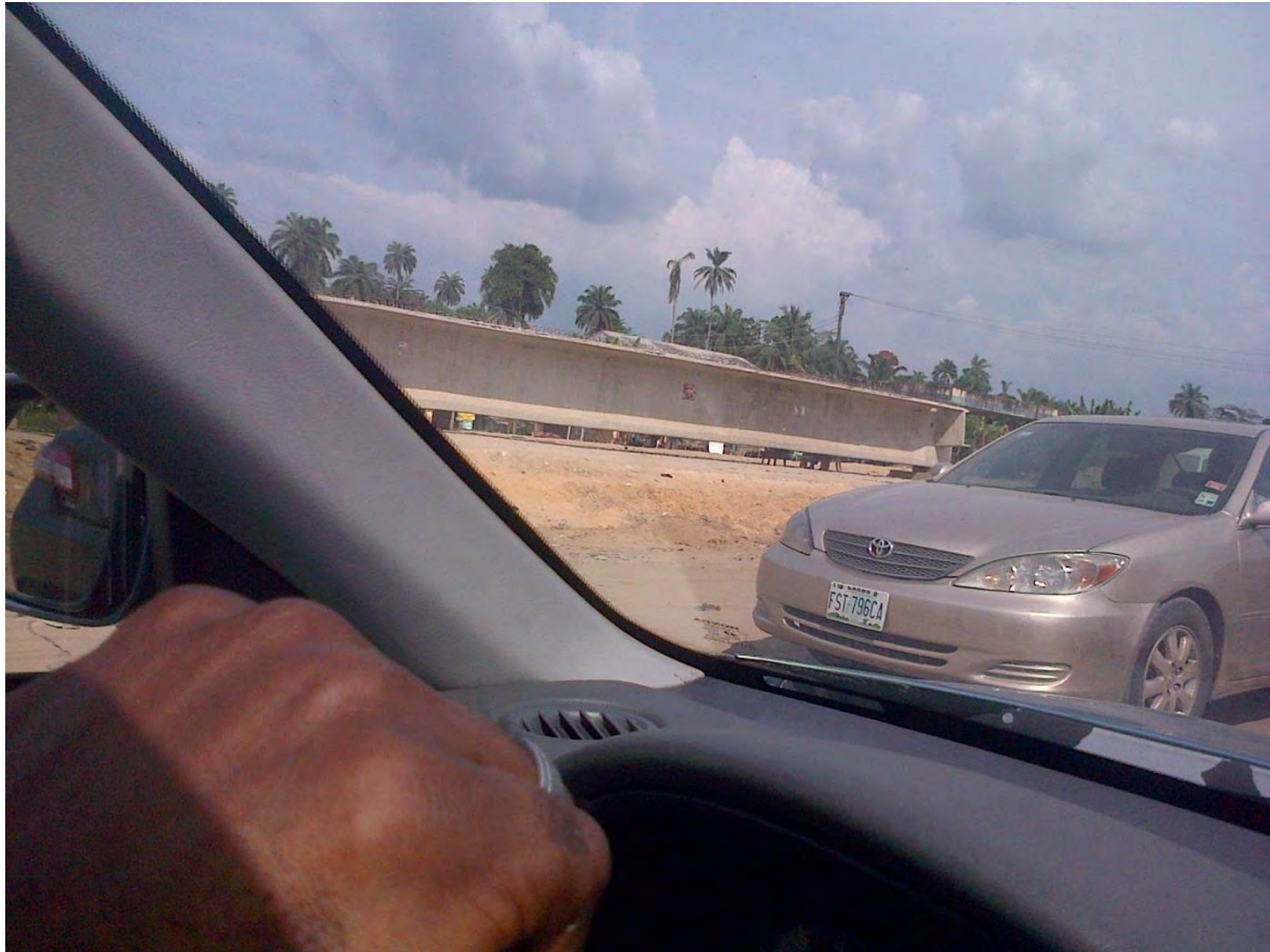
A federal government road project on a major road linking parts of Balyelsa State, November 2014.
