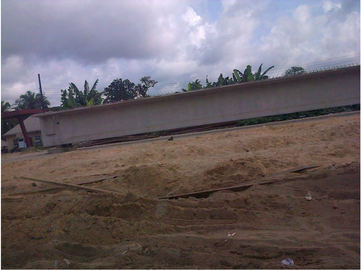
A road project under construction in Port Harcourt en route to Balyelsa State, November 2014.
