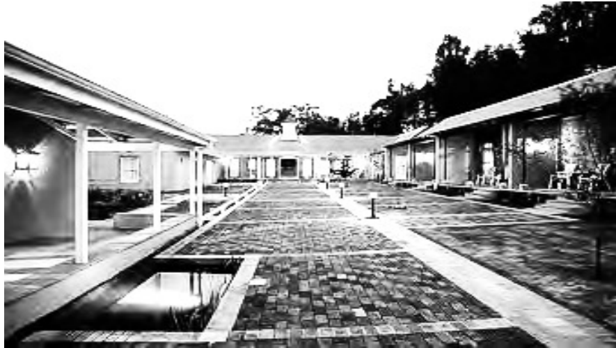
Figure 31 (above): The centralized courtyard demarcated by mixed materials.
