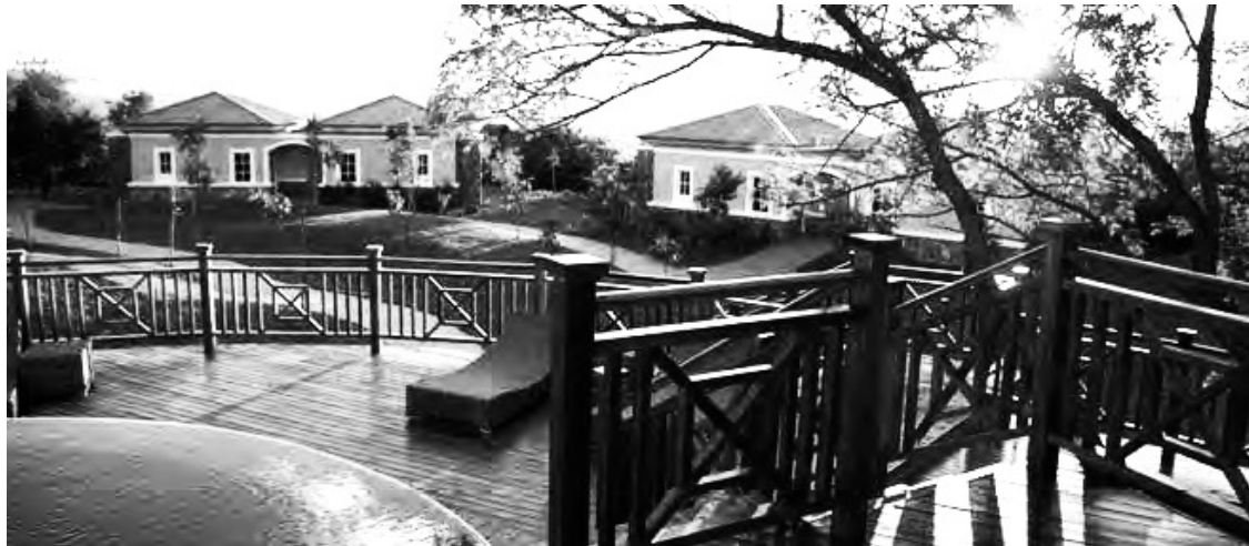
Figure 2 (above): A view of the spa, taken from opposing decks. ( www.africanpridehotels.com )
