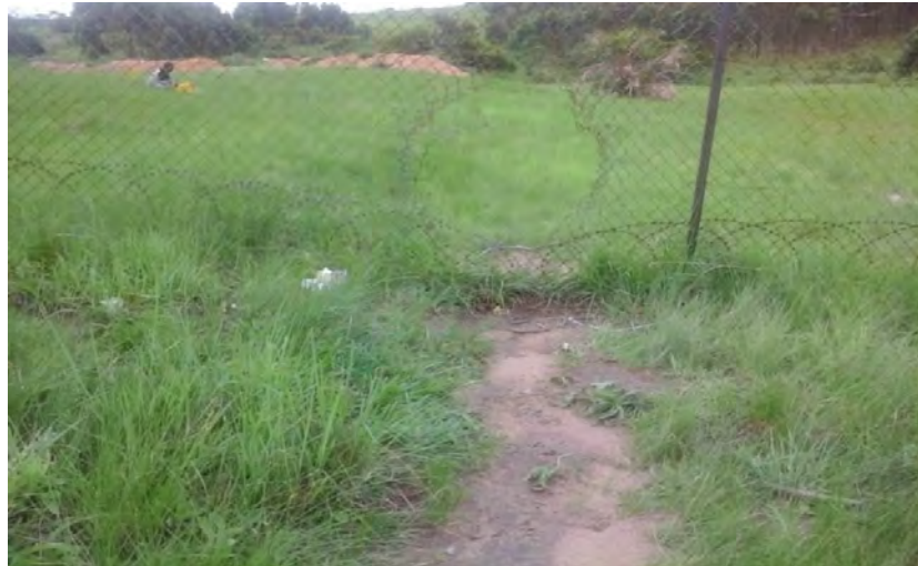
Figure 3.3: The hole in the school fence
