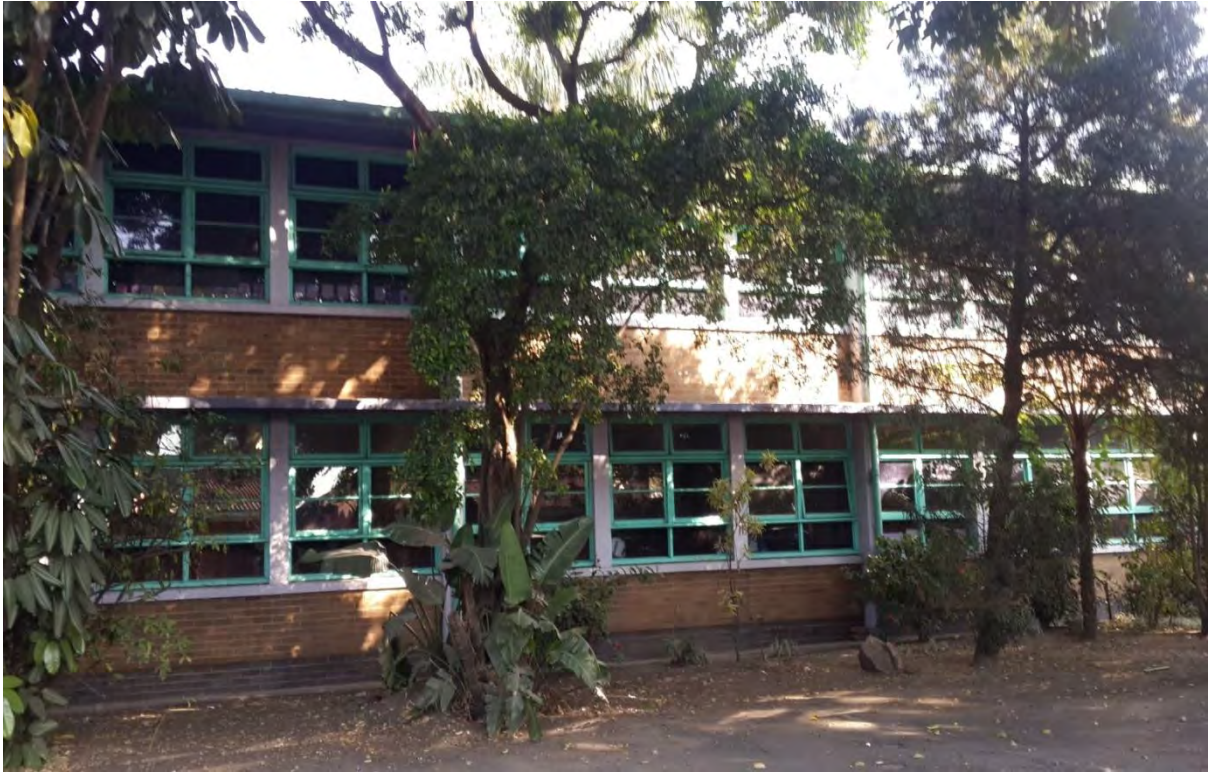
Figure 4.1: Aster Primary School building
