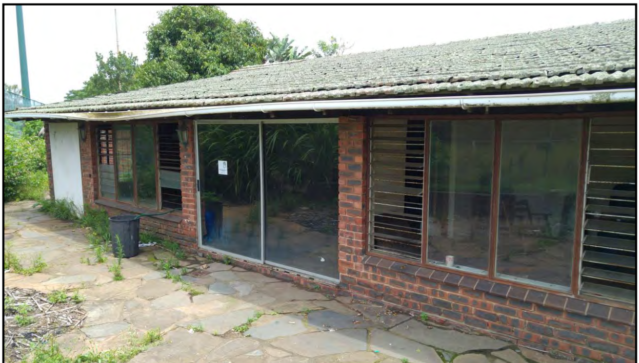
Plate 11: Abandoned Club House/Administration Offices
