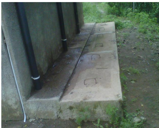
Figure 11: Closed cemented pits of VIP toilet in one of the schools
