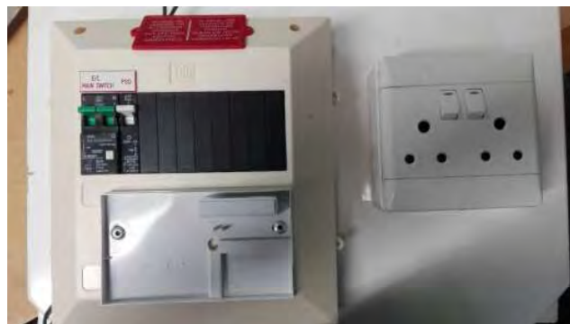
Figure 5-2: The 20 A ready-board
