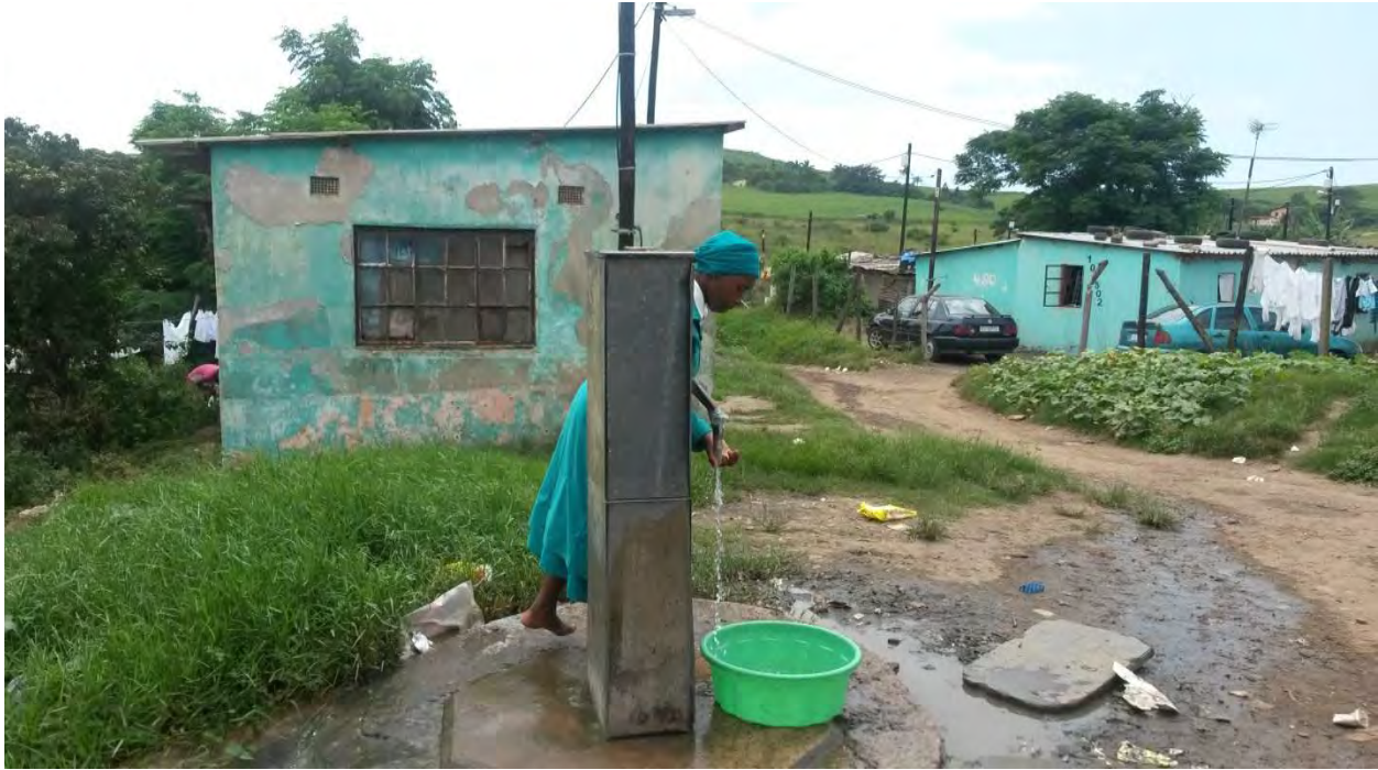
Figure 2: A water standpipe in Magwaveni informal settlement providing safe and clean drinking water to households.
