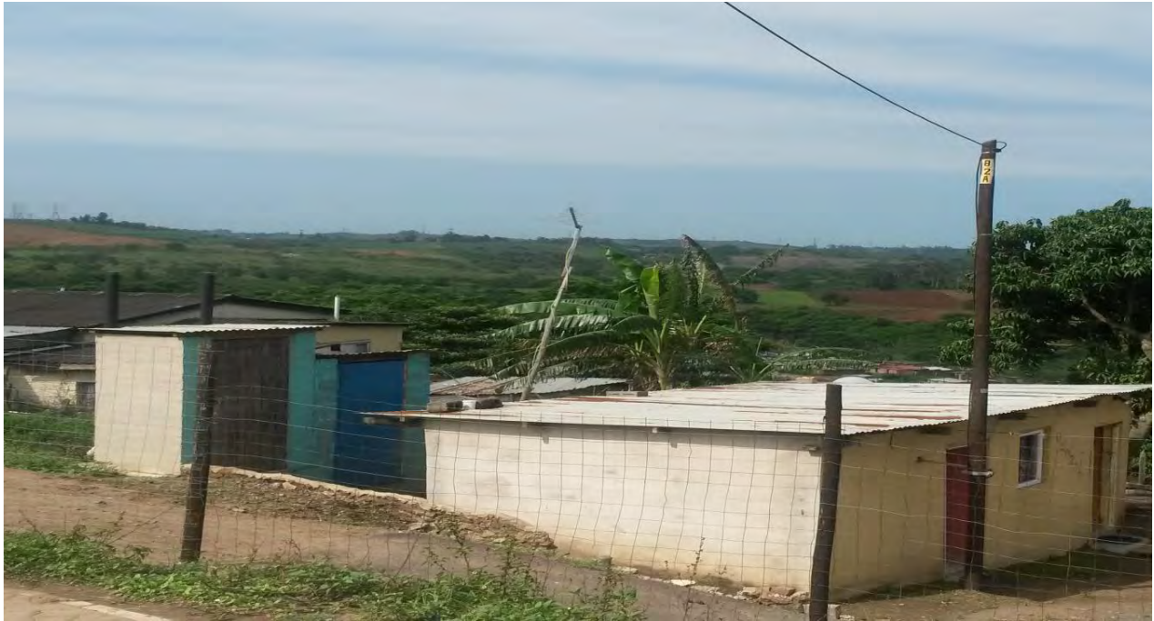
Figure 5: An informal dwelling with a VIP toilet in Redcliffe.
