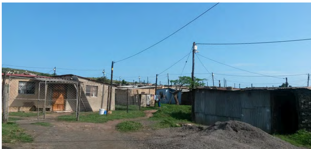
Figure 6: Informal houses connected with electricity in Magwaveni settlement.
