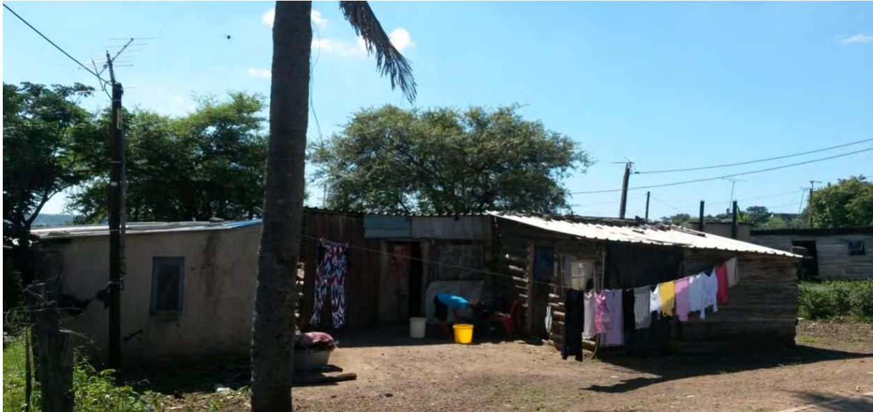
Figure 1: A typical informal dwelling unit in Redcliffe being gradually improved by the owner from a corrugated iron and wood structure to brick and mortar through sweat equity and savings after the provision of services.
