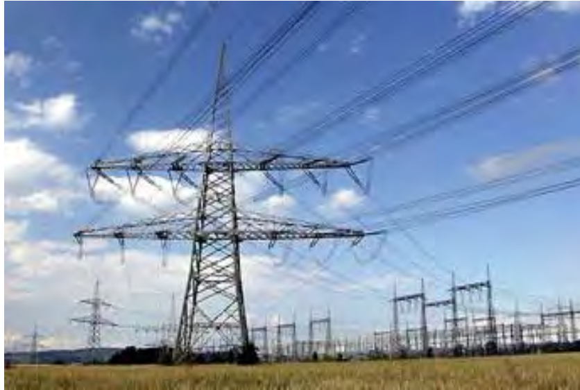
Figure 1-5: Power transmission line
