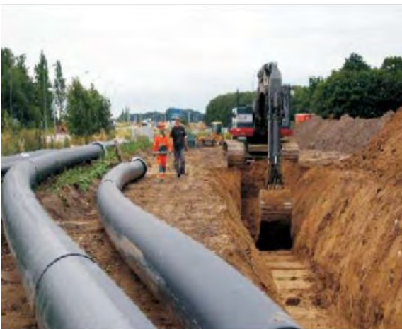
HDPE water pipes
